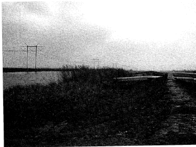
Figure 2. Facing west –Lake Cataouatche Levee with the Outer Cataouatche Canal on the flood side (to the left). The existing pipeline is going up and over the existing, non-upgraded levee.
